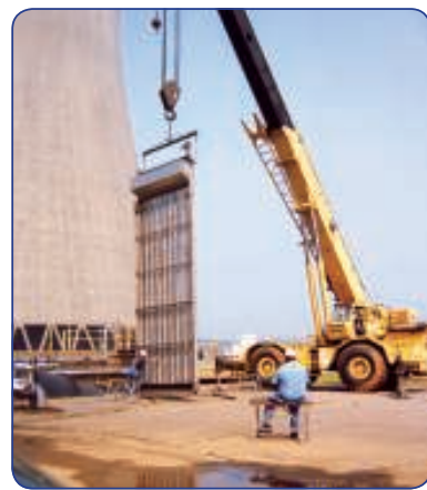
Traveling screens avoid the problems associated with cleaning fixed screens
