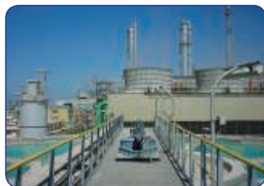
Softening with lime, shown here, is one of many treatment options offered by Ovivo
